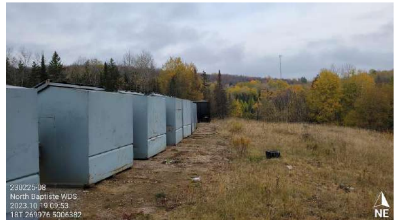
Photo 28: Vegetation growth on cap – October 19, 2023
