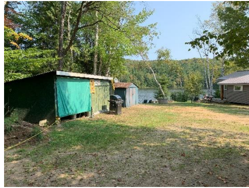
Photo 4. Existing garage and metal shed to be removed (September 12th, 2024).
