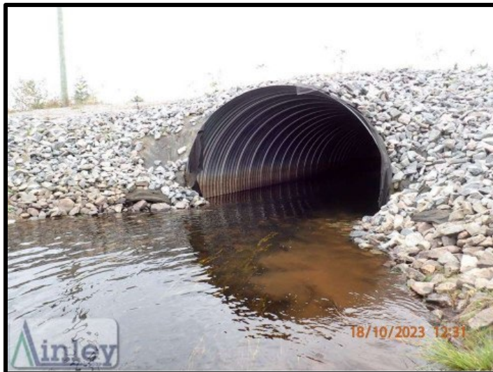
William Lake Road Culvert (BCI = 94.6 Very Good)
