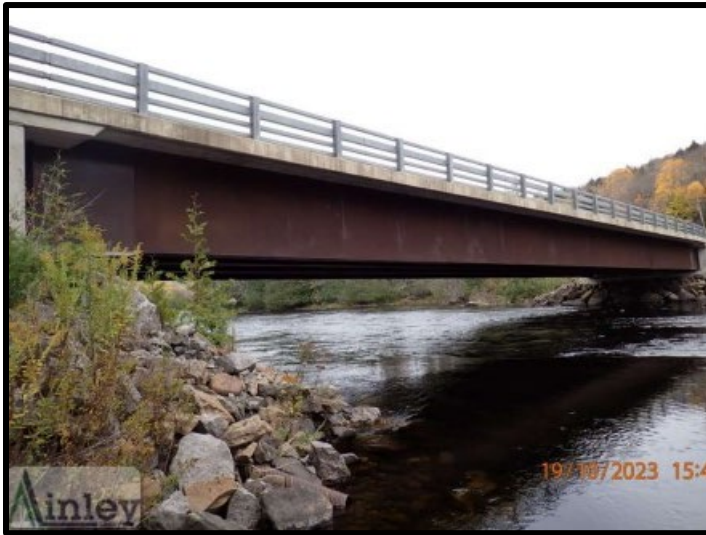
Siberia Road Bridge (BCI = 73.5 Good)
