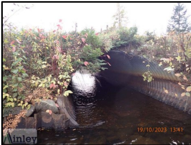
South Papineau Lake Road Culvert (BCI = 45.3 Fair)
