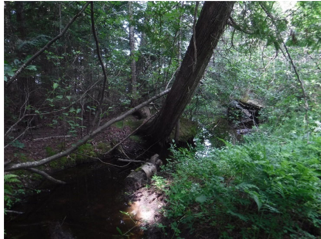
Photo 4 – Site Conditions of Watercourse Near Cottage 2. View Looking Southwest Towards Papineau Lake.
