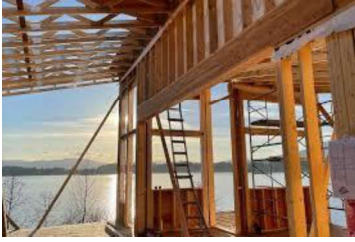
Waterfront construction site.
