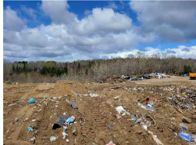
Photo 4: Cover material being added to active landfilling area – May 2, 2023
