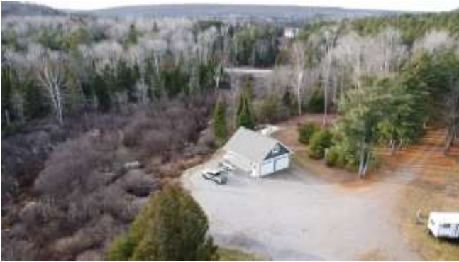
Photo 3. The existing garage and adjacent Papineau Creek wetland (November 15, 2023).
