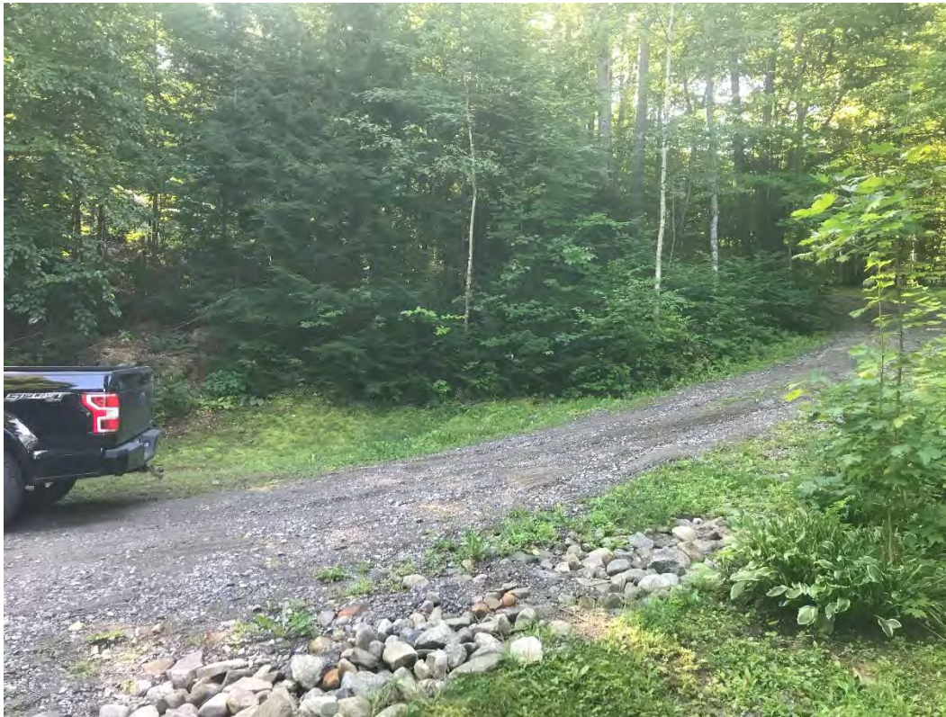
Photo 5 – Driveway at 3248 Papineau Lake Road with existing “French Drain” (August 24, 2021).
