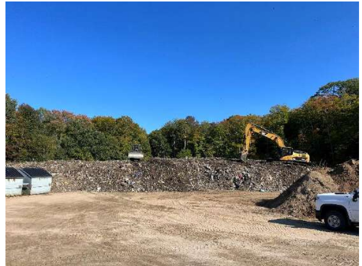
Photo 24: FBAL excavation – September 21, 2023
