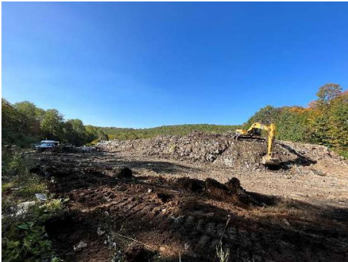
Photo 23: FBAL excavation – September 21, 2023
