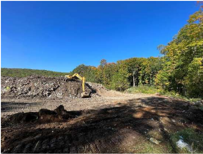
Photo 21: FBAL excavation – September 21, 2023
