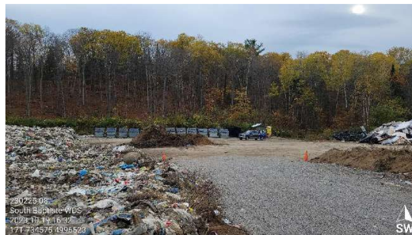
Photo 32: Landfilling site, facing southwest – October 19, 2023
