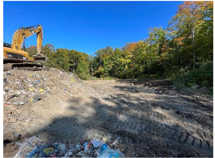
Photo 22: FBAL excavation – September 21, 2023
