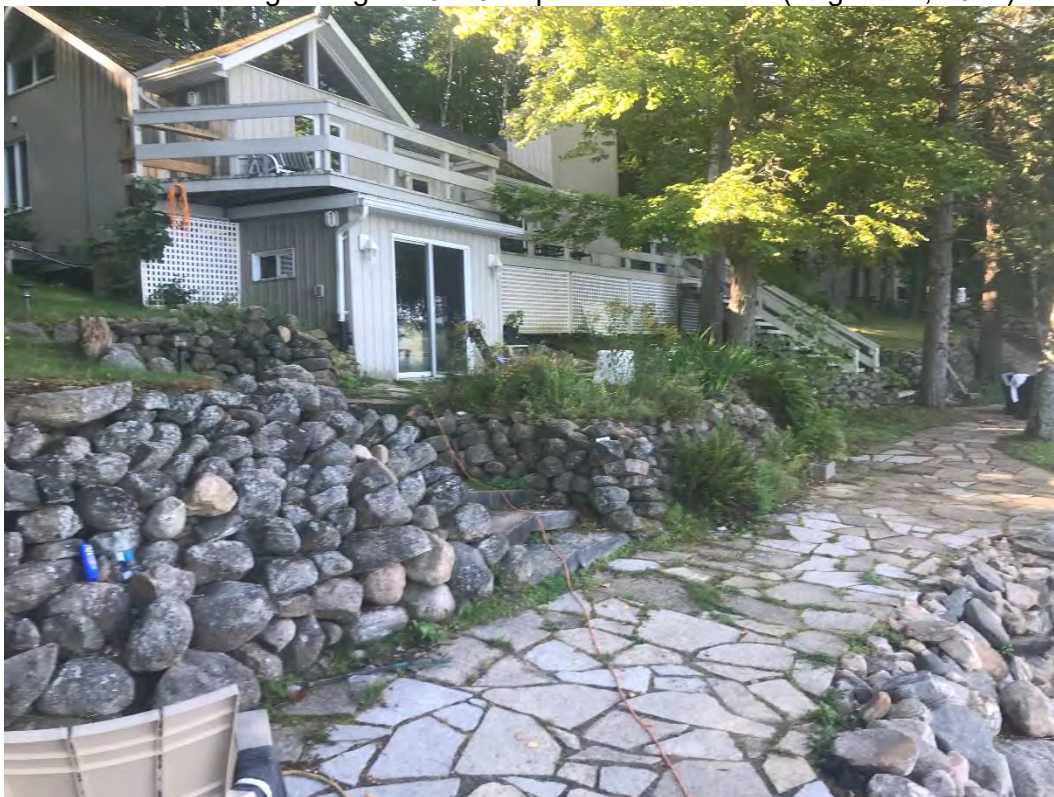
Photo 2 – Existing cottage at 3248 Papineau Lake Road (August 24, 2021).
