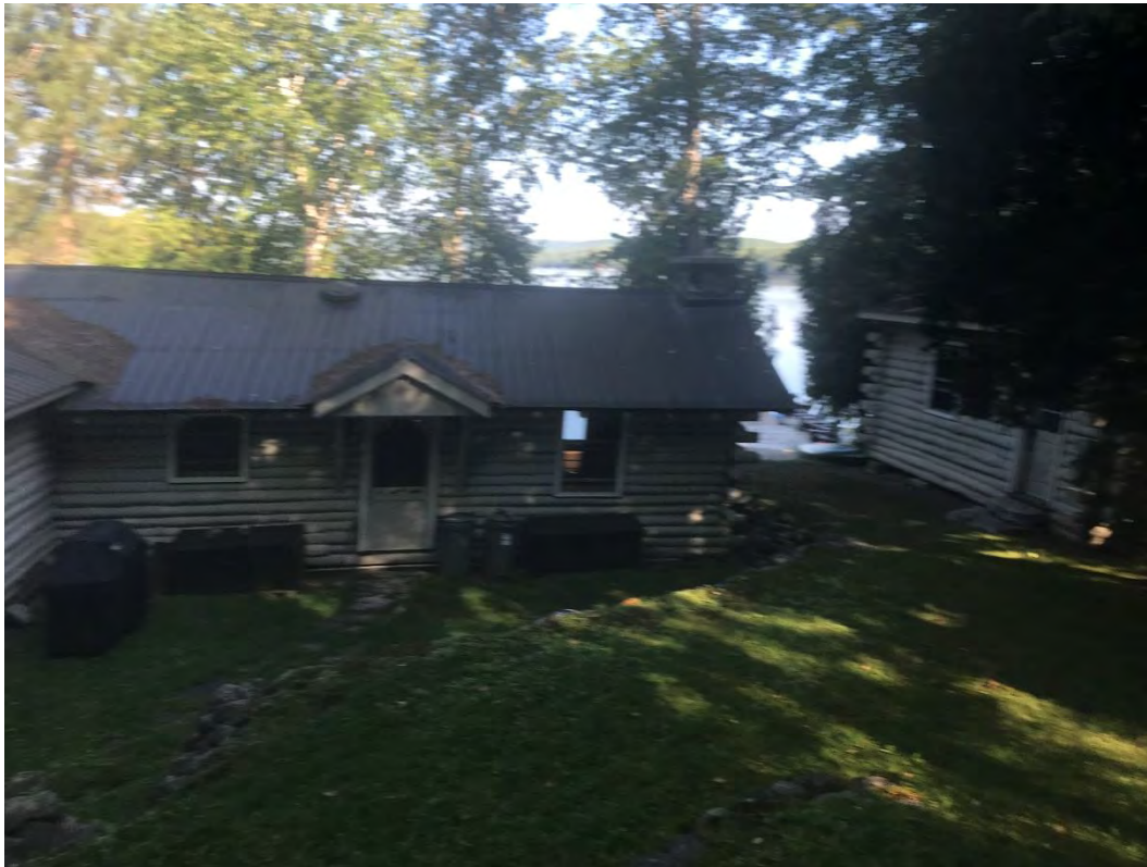
Photo 1 – Existing cottage at 3240 Papineau Lake Road (August 24, 2021).
