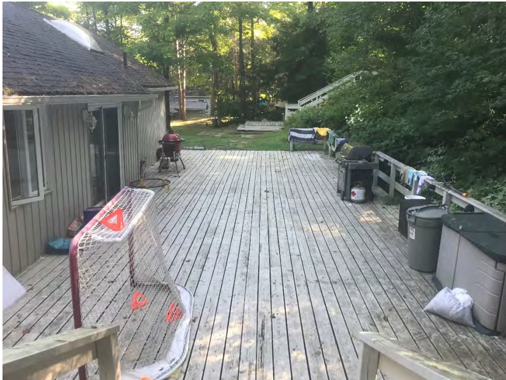
Photo 4 – Existing deck at rear of 3248 Papineau Lake Road building (August 24, 2021).
