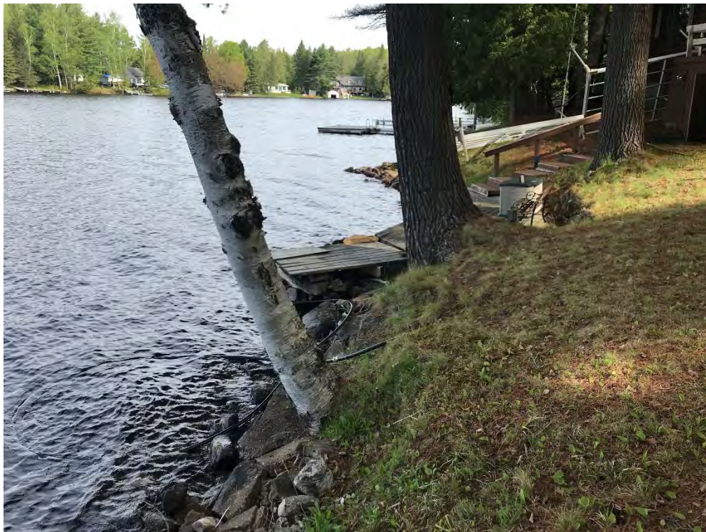
Photo 2 – Existing shoreline area looking north (May 17, 2024).
