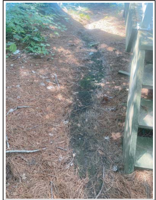
Photo B: minor erosion down the west side of the existing cottage.
