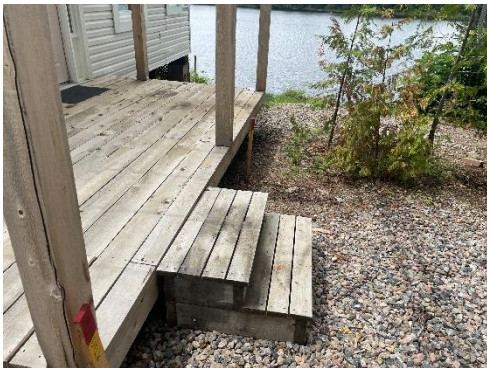
Photo 3. Existing deck adjacent to cottage (July 25th, 2024).
