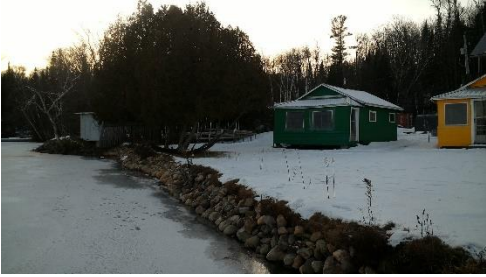
Photo 1. Existing conditions along shoreline cottages in the background (December 14, 2023).
