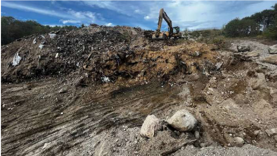
Photo 19: After FBAL excavation – September 15, 2023.
