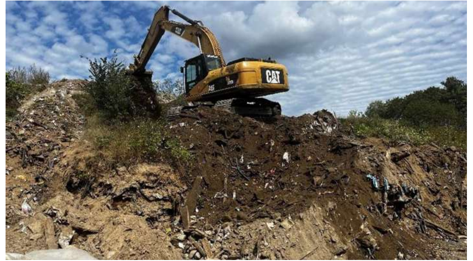
Photo 18: FBAL excavation – September 13, 2023.
