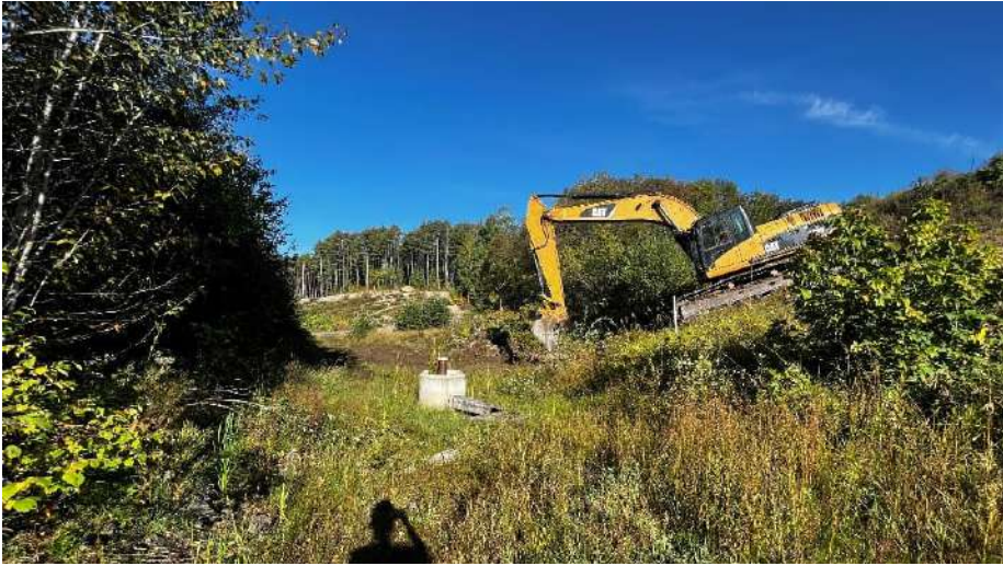
Photo 17: Before FBAL excavation – September 11, 2023.
